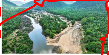
Karnataka is planning a dam over the Cauvery at Mekedatu to meet the drinking water needs of Bengaluru. B. JOTHI RAMALINGAM
