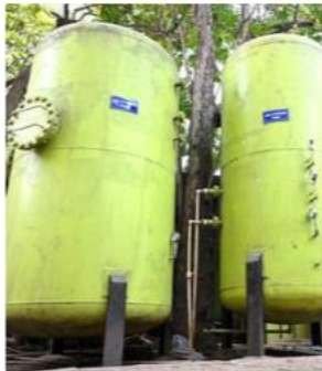
A biogas Plant at Bengaluru in the State of Karnataka.
