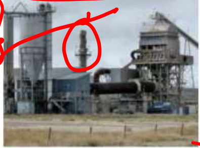
A rotary kiln is visible as the rust-coloured horizontal tube at the centre in this image of a cement plant in the U.S. GREG GOEBEL (CC BY-SA)
