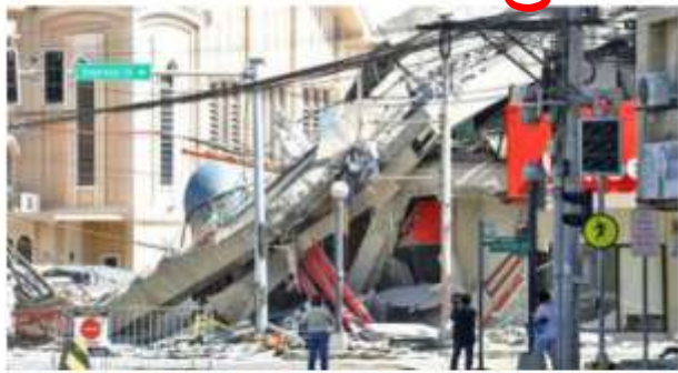
Rubbled remains: A damaged building seen in General Santos, Philippines, following a magnitude 7.8 quake on Monday. AP
